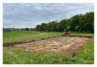
We are in a very exciting phase of the build on 'The Hive'. With phase one fully complete (the site prep) we have now started phase 2 (the building of the Pavilion) this week. The foundations are now complete ahead of the building's arrival which will go in during the summer break.
